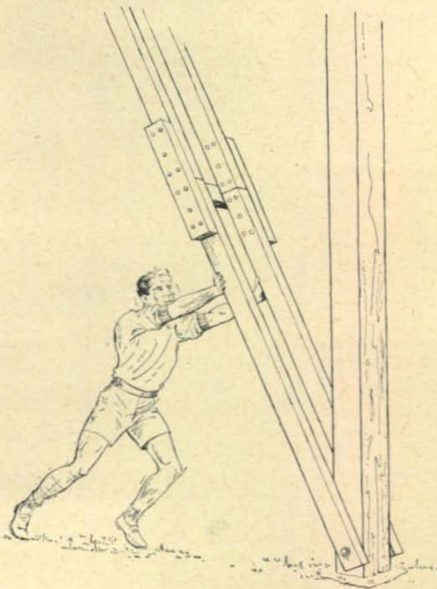
Fig. 5—Method of walking the mast up after inserting the base pin. Perhaps a few cans of liquid refreshment might get a few helpers.
